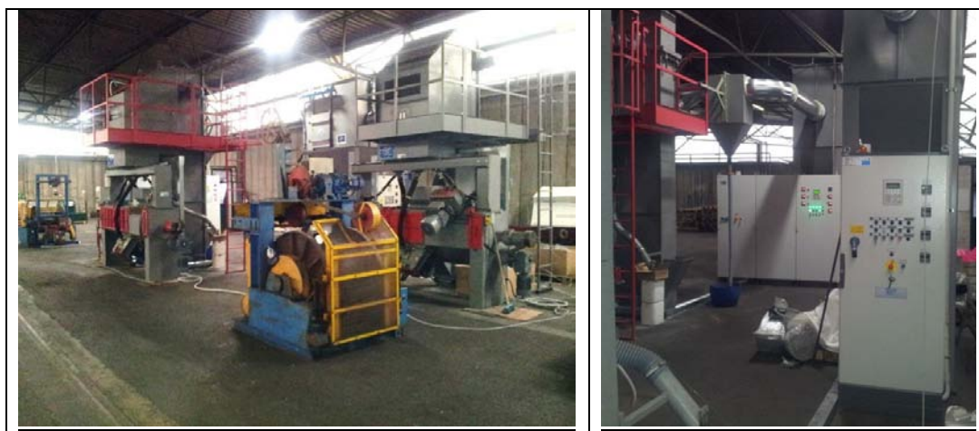
Fig. 4: Final Pilot Line
